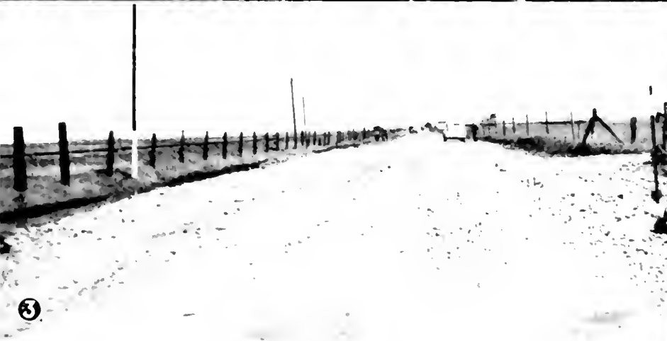
Some maintenance jobs. 1. Section of State Highway surface in Santa Barbara County, destroyed by military traffic. 2. Damaged surface of State Highway in Imperial County by hauling operations due to war emergency. 3. Damaged surface of State Highway in Merced County by contractors equipment hauling to defense project. 4. Section of State Highway surface in San Bernardino County damaged during military maneuvers.
